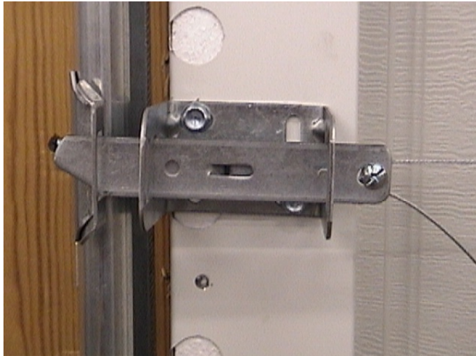
Installed Snap Latch Lock FIGURE 11
